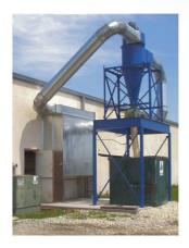
**Cyclotron.** High efficiency cyclone separator provides reliable, low maintenance operation with direct drive, backward inclined airfoil blowers on the clean side of the cyclone.
