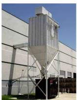
**Bagtron.** Pulse jet baghouse dust collector keeps up with the most demanding jobs, providing online cleaning for continuous-duty operation.
