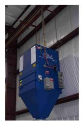
Flowtron AC. This unit is used in areas where source capture of welding smoke is not feasible. Its high-powered capture velocity and automatic filter cleaning make the free-hanging industrial air cleaner an outstanding performer for weld smoke. The only regular maintenance required is the emptying of the barrel located on the floor. Optional hopper allows 4 to 10 units to be hooked together for automatic emptying of the hopper.
